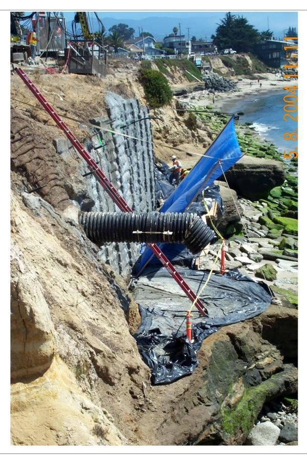
This illustration depicts the construction method that would be used to install soil nails for the East Cliff Drive project. Much of the drill work would be done from the edge of the blufftop. Additionally, in the final stages of construction, workers suspended from the blufftop would apply the shotcrete layers.
